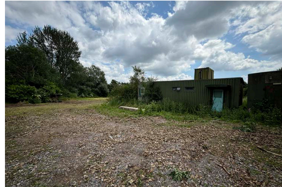
2 Existing site buildings and hardstanding area
