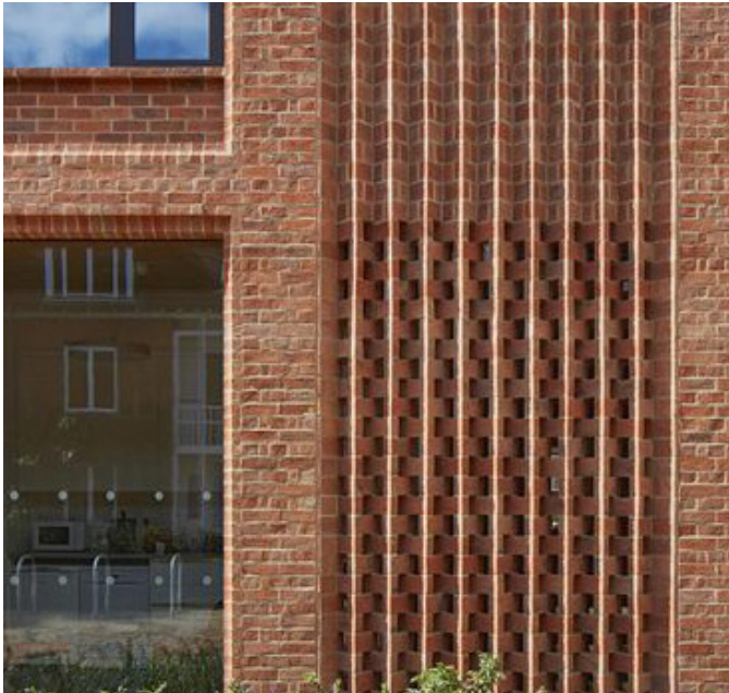
Brick detail, decorative projecting brickwork
